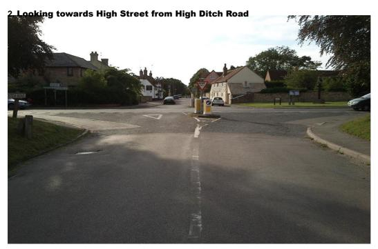
Note the position of the centre island. For some reason the island at the High Ditch Road junction is offset towards Horningsea and this makes it more diff cult for motorists from Horningsea Road to get a good view past the parked cars in High Ditch Road. The width of High Ditch Road is 6 metres wide, which is narrower than the High Street's 8.5 metres width.
